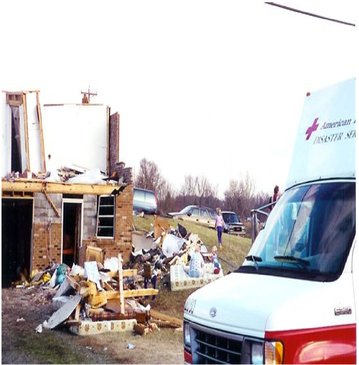
January 1999 Tornado Damage
