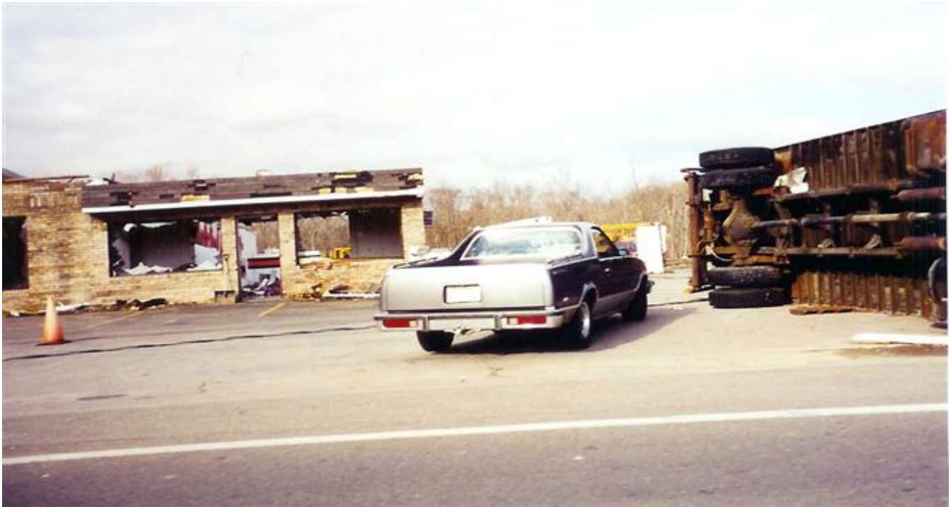
January 1999 Tornado Damage
