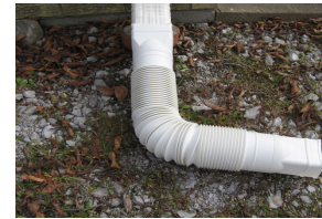
Downspout leading directly into an underground pipe is replaced by a plastic flexible downspout extension available at hardware stores.
