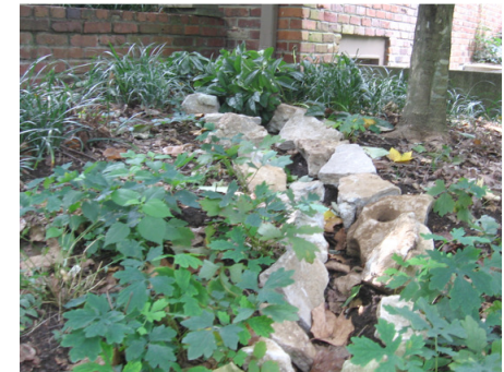
A dry creek bed made with stone carries the rainwater from the downspout to the rain garden area.
