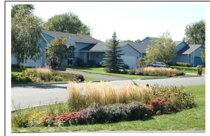
Rain gardens in Burnsville, MN. Photos courtesy of Barr Engineering and City of Burnsville, MN: Fred Rozumalski, Landscape Architect and Kurt Leuthod, Civil Engineer
