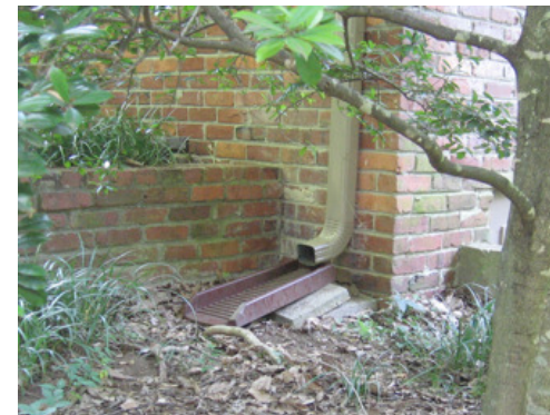
Run-off from the downspout was pooling next to the foundation. This was a perfect opportunity for a rain garden
